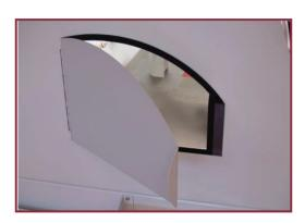
Make sure that the hatch is closed as soon as possible after openings. It is not spring loaded.
